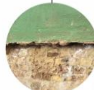
Existing coloured render and brick
